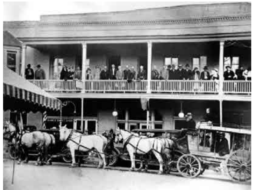
The Franco-American Hotel has stood at the intersection of Fourth and Miner Streets for over 150 years. It began as a small establishment in 1855 and grew with the town. The hotel became a regular stop for stagecoaches arriving in Yreka. It was the crossroads of the community. Today the building looks much the same as it does in this picture, but it is no longer a hotel.
