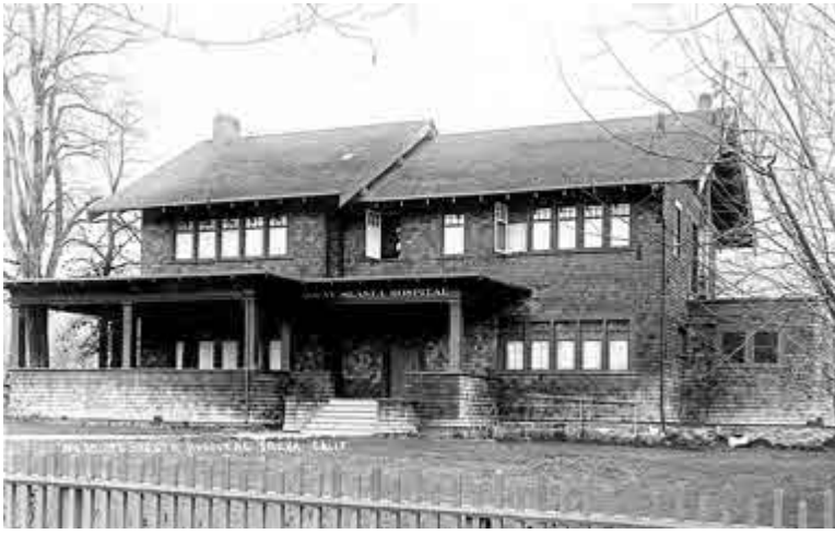
The Mt. Shasta Hospital building in Yreka as viewed in 1914. Photo from the Claudia East Collection.
