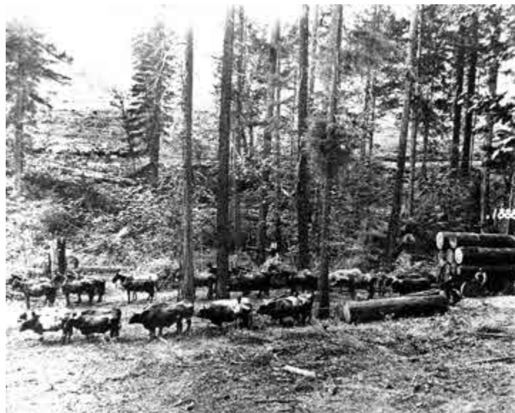
This 1888 photo shows lumbering activity of the Scott Mill - one of several mills near Mott. The amount of milled lumber produced at Mott is amazing considering the methods used at that time. Photo submitted by Ron McCloud.
