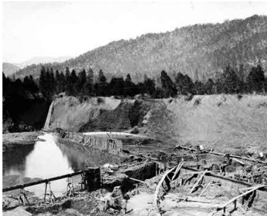
PHOTO: Hydraulic mining operation. Courtesy Fort Jones Museum.
