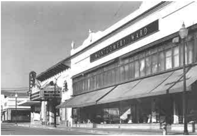
The Montgomery Wards Building as seen in 1941, with the Broadway Theatre sporting its original Moorish Design. Photo Courtesy Claudia East.
