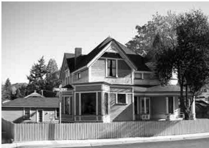
Parr Steel House on Third Street, Yreka. Photo courtesy Claudia East
