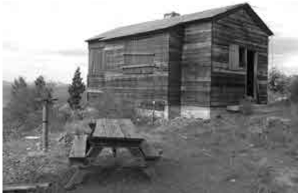
Photo of the cabin that sits below the tower.
