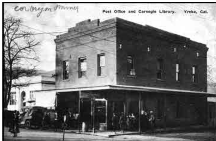
Stimmel Building when it was the Post Office, circa 1920 Photo courtesy Claudia East Collection.
