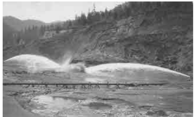
Photo: Hydraulic mining was used to wash away hillsides after the easy gold played out. A Schueffler photo c. 1915. Courtesy Gail Jenner Collection.
