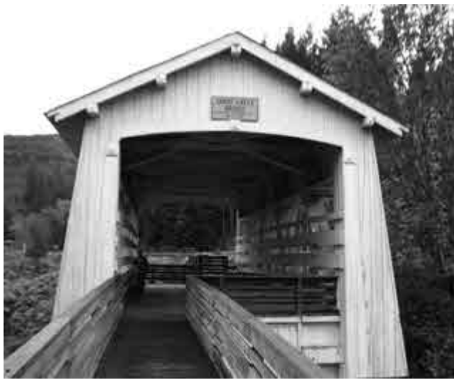
Photo of Sandy Creek Covered Bridge taken in 2011 by M.Fain.
