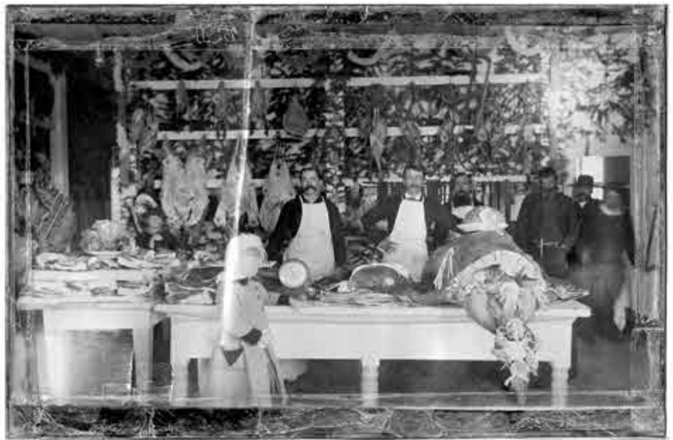
Historic Photo inside Herzog City Meat Market. The metal racks and hooks behind them are still in use in the new Miner Street Meat Market.
