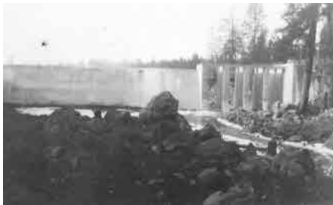
Photo below: Front side of Gilchrist mill pond dam, 1938.
