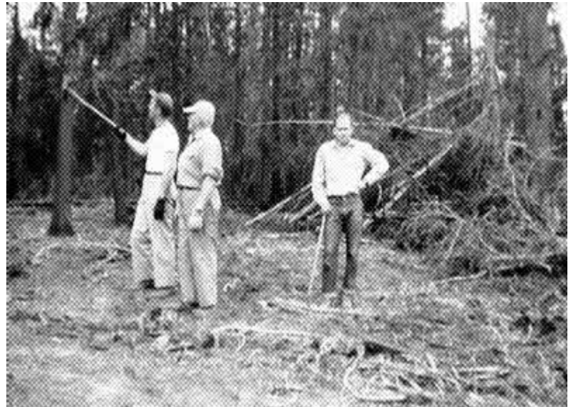
Crescent Community Club site clearing. Photo submitted by John C. Driscoll.
