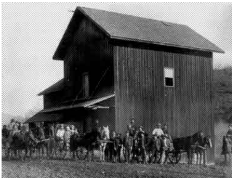
Historic Photo of Butte Creek Flour Mill circa 1890 (above) and the devastating fire photo (below right) submitted by Bill Wensrich.
